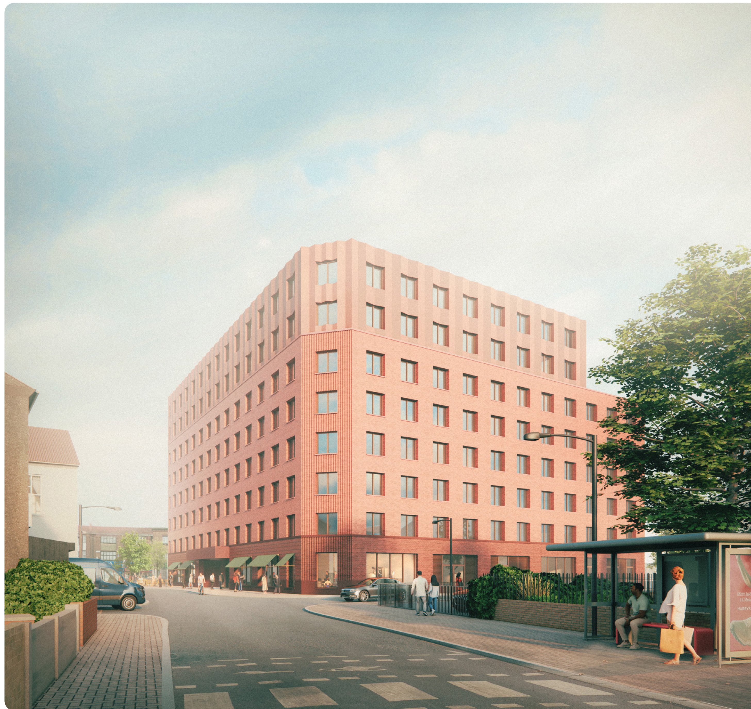
View from Willow Walk towards High Street
